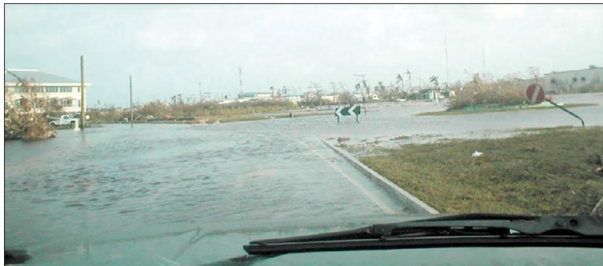
► Flooded roundabout during Hurricane Ivan 2004
