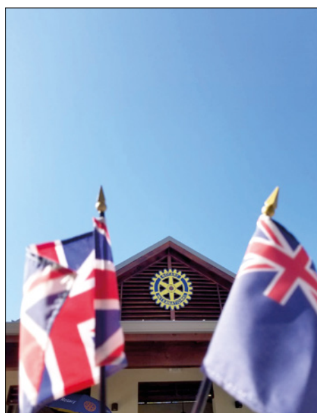
▶ Rotary Schoolhouse With Flags in Foreground
