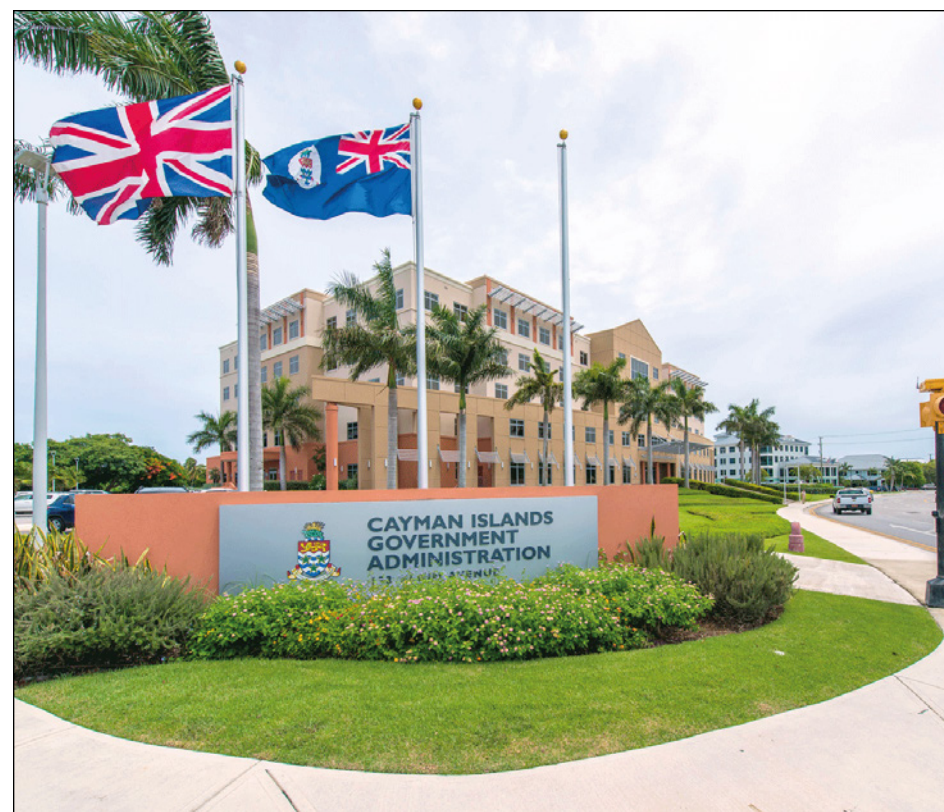
► Cayman Islands Government Administration Building
