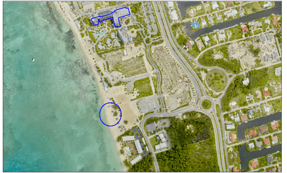
► Aerial photo of the area under works
