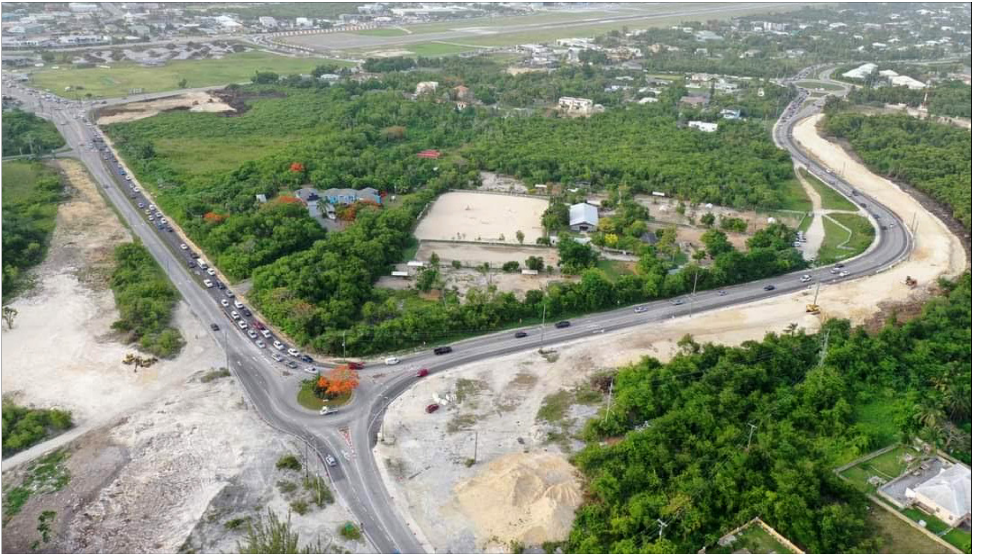
► Aerial view of the progress on LPH works – July 2022
