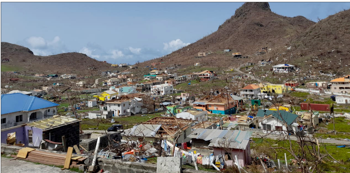
► This image shows the scale of damage on Union Island.
