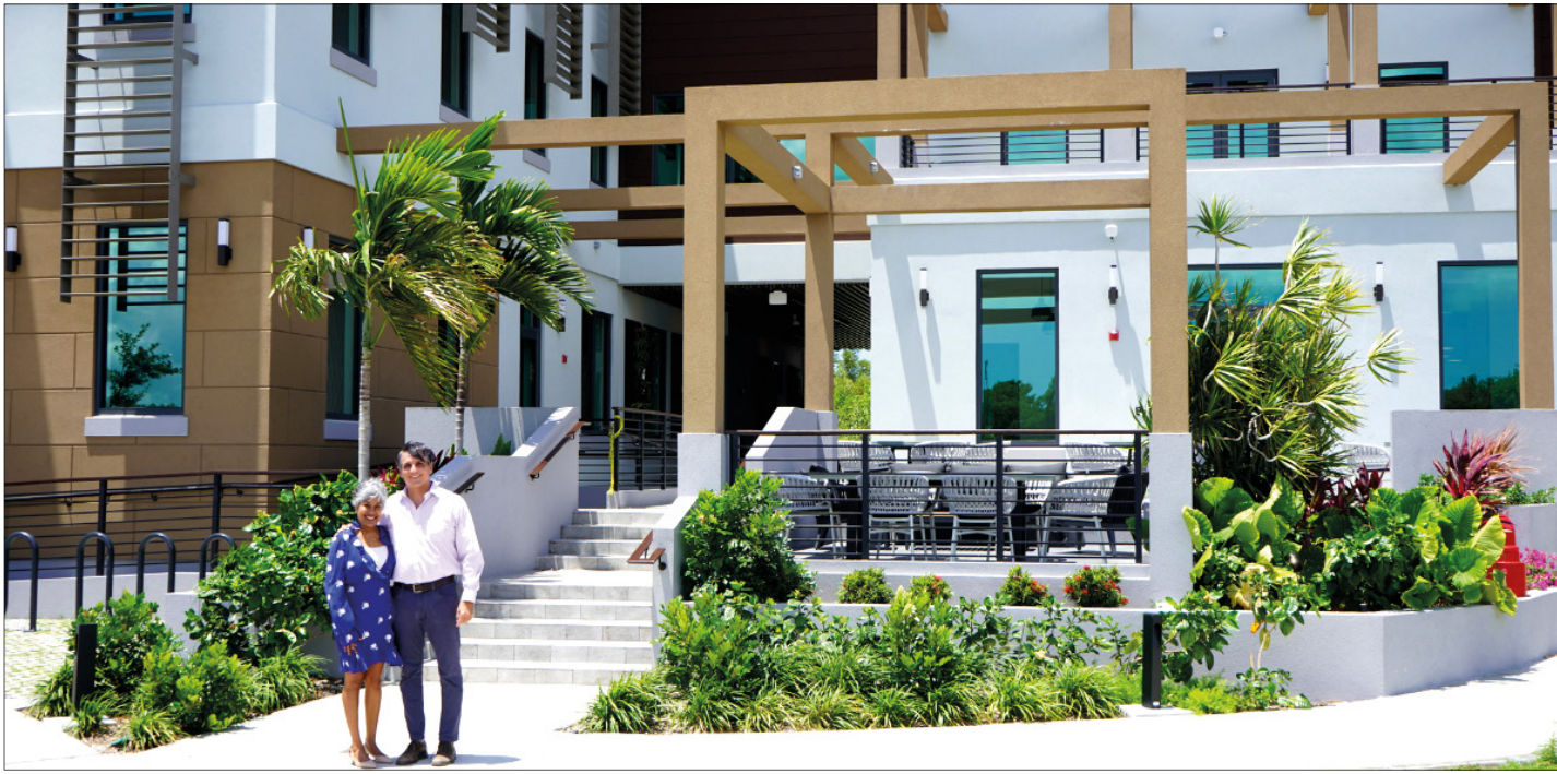
► Marla Dukharan and Charlie Kirkconnell stand in front of CEC's new facilities Signal House
