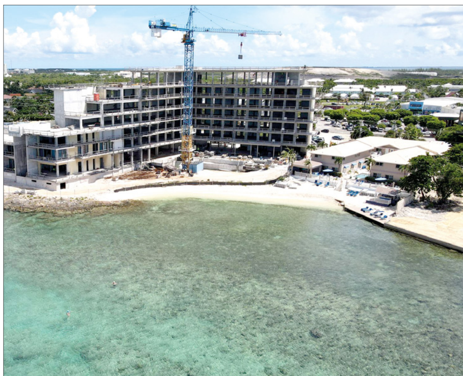
► Construction at Kailani Grand Cayman reaching the seventh floor
