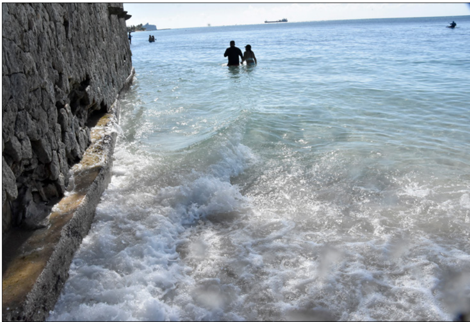
► There is literally no beach left in some places. This photo is taken from the top of the beach, just north of where Royal Palms used to be
