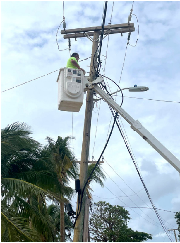
► Utilities technician repairing power line. Photo credit: HMCI
