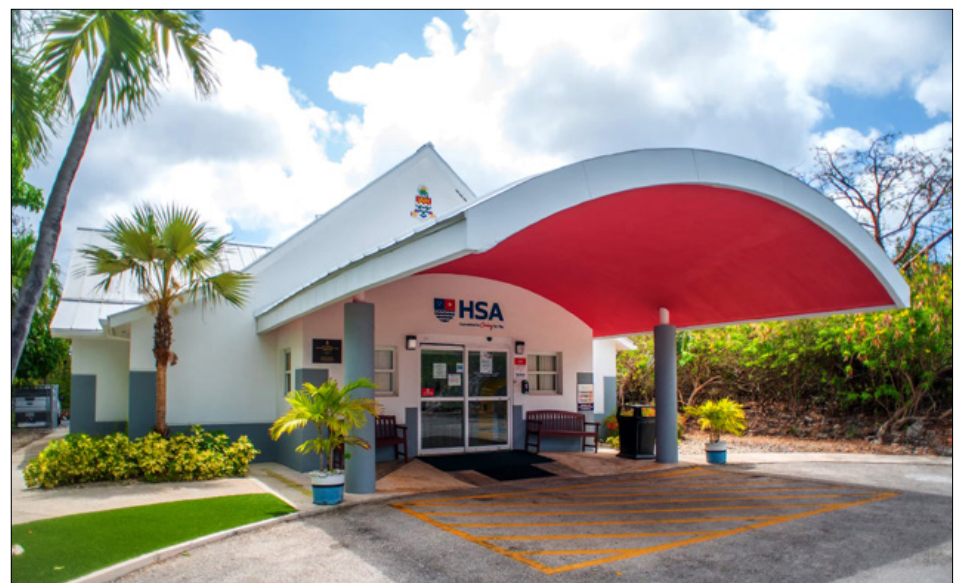
► North Side Health Centre
